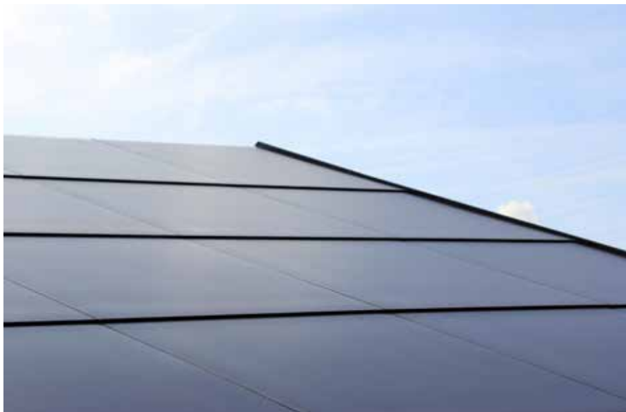
Frameless PV Module with thermally toughened 2 mm thin double glass
