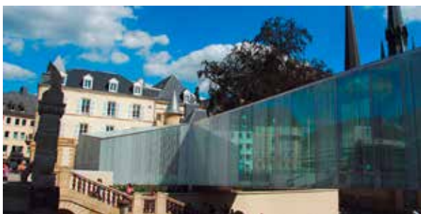
GLAZED FOOTBRIDGE - LUXEMBOURG CITY HALL - Twenty five meters long glass walkway connecting two buildings of the Luxembourg City Hall and creating a reception room for marriage ceremonies.
