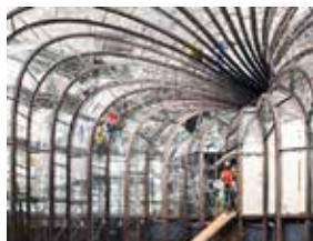
MANTA GLASSHOUSE – Bombay Sapphire. Two glasshouses have been designed by Heatherwick studio for the new distillery and visitors centre of Bombay Sapphire in Laverstoke. The Glass houses structures are free-standing and are sitting in the water.
