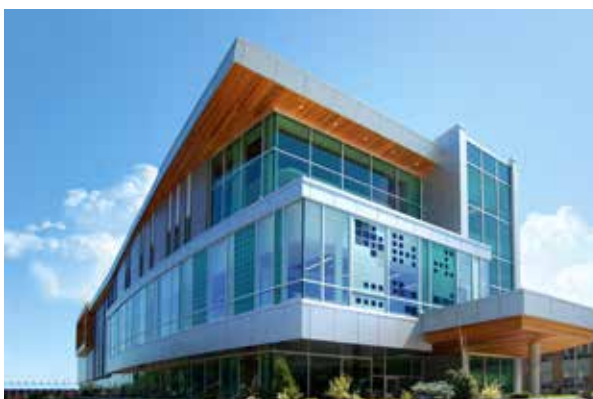
Application of facade decorated glass panels with integrated PV modules and heating
