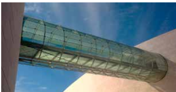
GLASS BRIDGE, CHAMPALIMAUD FOUNDATION. The glass bridge connects the two buildings in the complex. The bridge consists of a single section steel structure with a 22-meter longitude with a post-stressed net of cables along the bridge, in addition to a total of 12 vertical rings every 2 meters braced with compression elements.
