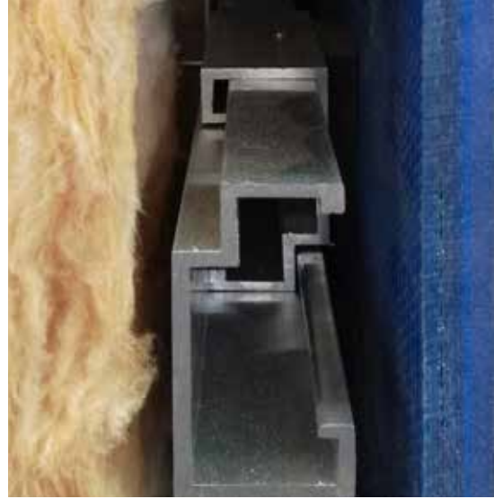
FKV-VH-Fassade (© Jan Wunsch) Ventilated façade with FRP (fibre-reinforced polymer) (© Jan Wunsch)
