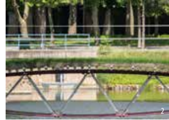
(1) Glass Swing build out of glass struts (2) Glass struts applied in pedestrian bridge at TU Delft campus.
