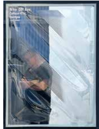
Nike Flagship Façade – Carved and Slumped Insulating Glass Units
