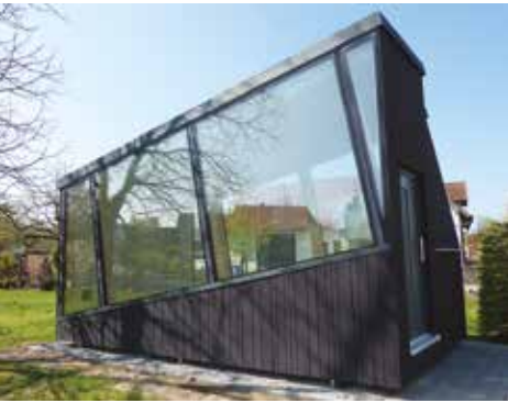
Pilotbau Holz-Glas- Verbundfassade (© Gump & Maier GmbH) Test construction timber-glass composite façade (© Gump & Maier GmbH)
