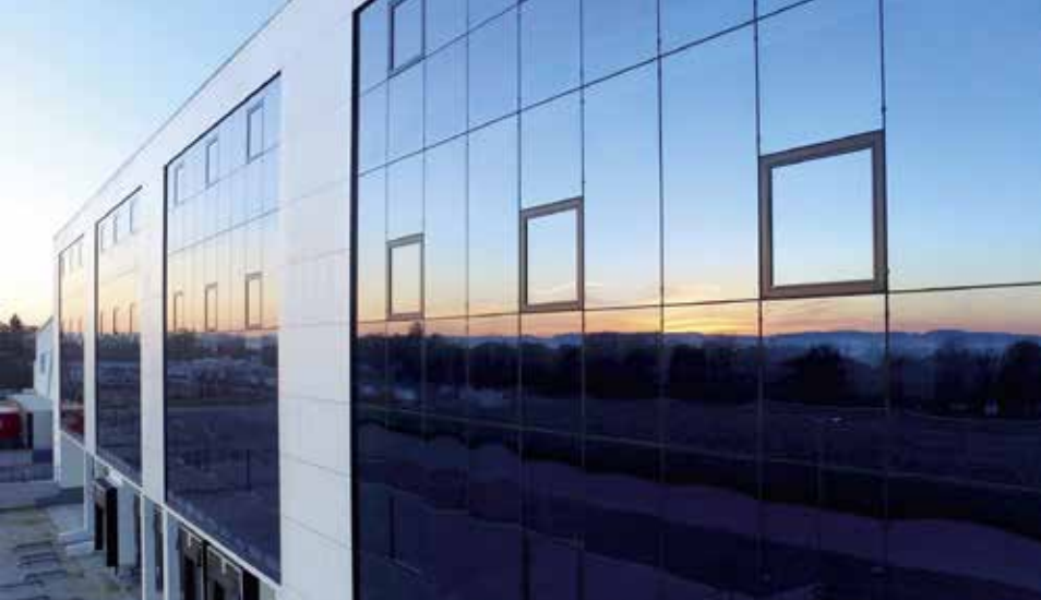
Holz-Glas-Verbundfassade in Fridolfing (© OTTO-CHEMIE) Timber-glass composite elements in use: façade of a logistic centre in Fridolfing (© OTTO-CHEMIE)
